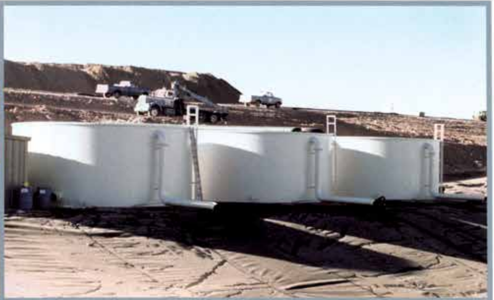
Field erected slurry tanks for a mine in Northern Nevada. ➤
