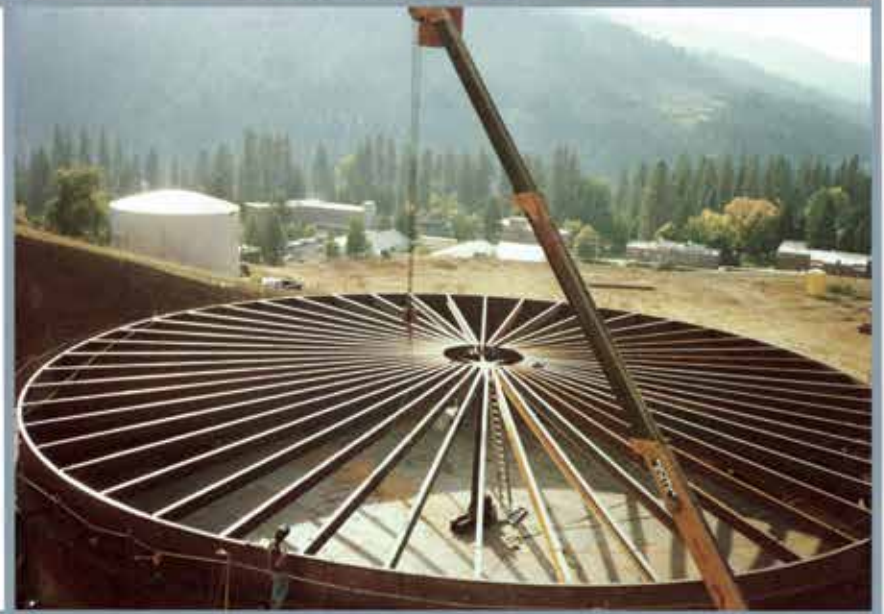
Field erection of a one million gal. capacity tank and roof in Northern Idaho. ➤
