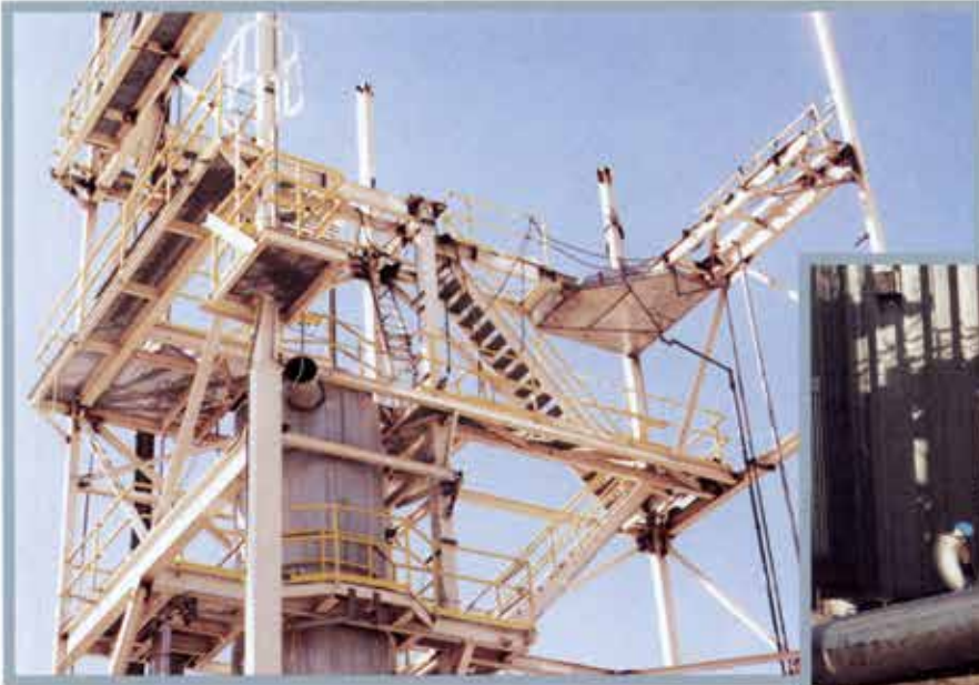
Dismantle in New Mexico, transport and install customer's stainless steel evaporator plant for a Southern Idaho sugar processing plant.
