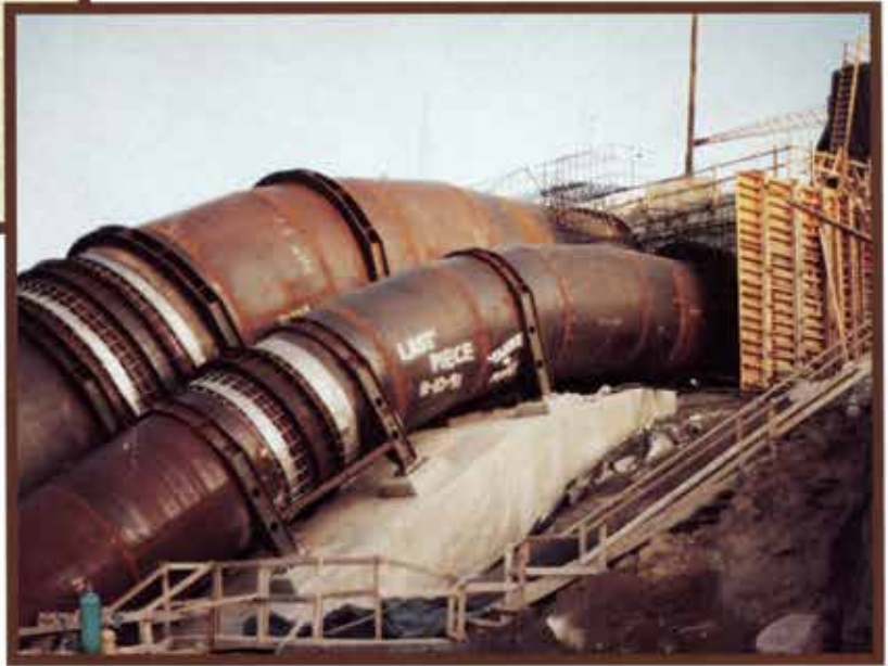
9 ft. dia. and 17 ft. dia. penstock fabrication, delivery and installation at Milner Dam in Southern Idaho.
