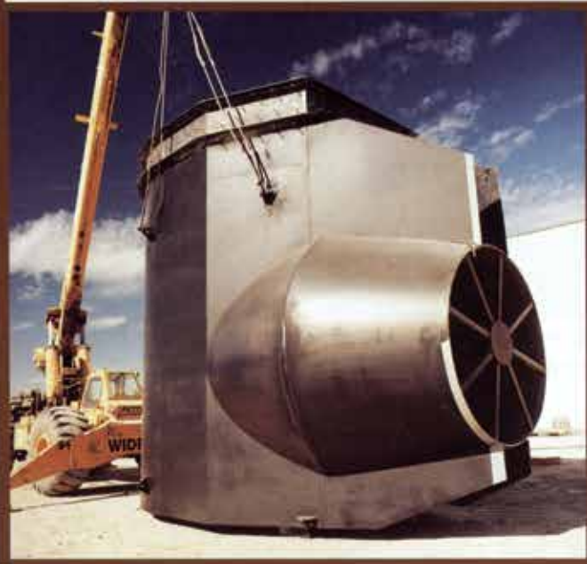
Pit liner for the Hazelton B and Wilson Lake Hydroelectric projects in Southern Idaho.
