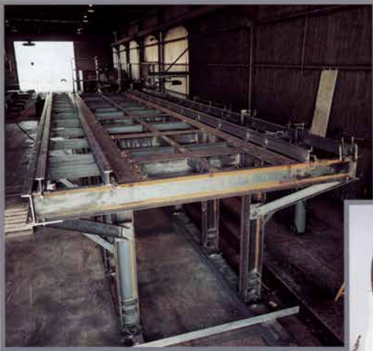
▶ Bolted structural steel platform for a mining operation in Indonesia.
